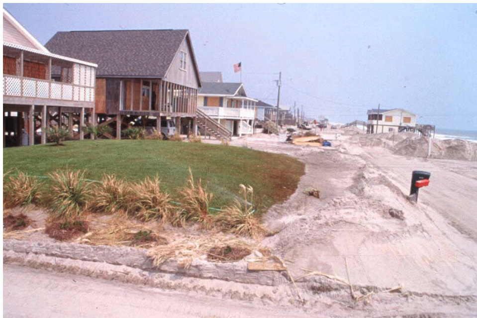
Figure 10: Second-row dune left after Hurricane Fran provided protection during Hurricanes Bonnie, Dennis and Floyd. Location North Topsail Beach after Hurricane Floyd.
